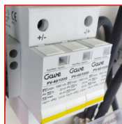
Surge protectors Phase connection on top and earth connection on bottom. Module end of life visual indication
